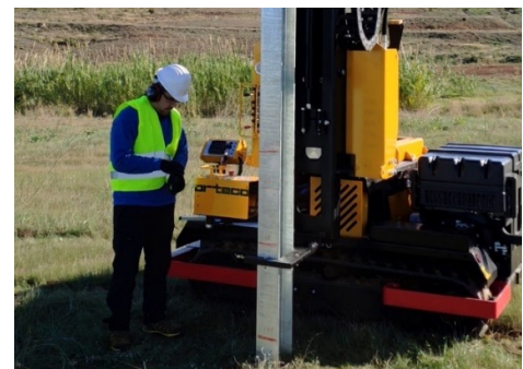
Figure 14 : Tracker Post Ramming Site
