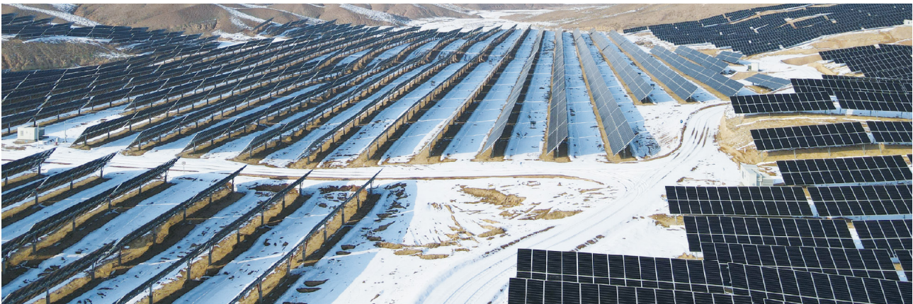
Figure 9 : Antai Ningxia Delivered Project Site
